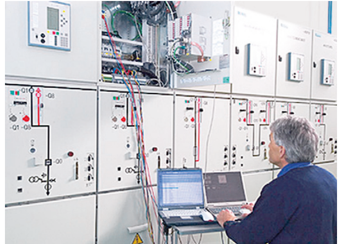
Fig. 2/32 Protection engineer at work
